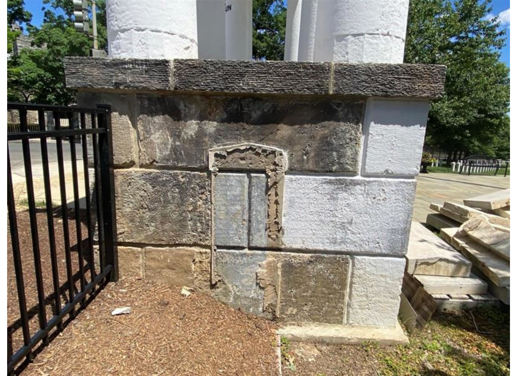
Detail view from inside SAHNC of the southern face of the Main Entrance Gate's stone base, where mortar remnants leave a ghosted outline of the southern wing wall (2024)
