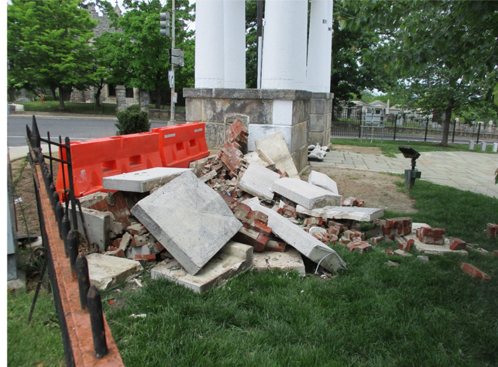
View from the Harewood Rd NW sidewalk adjacent the boundary fence looking north toward the SAHNC Main Entrance Gate southern wing wall after hit by vehicle. Note the case stone cladding panels and the exposed inner brick core (2024).
