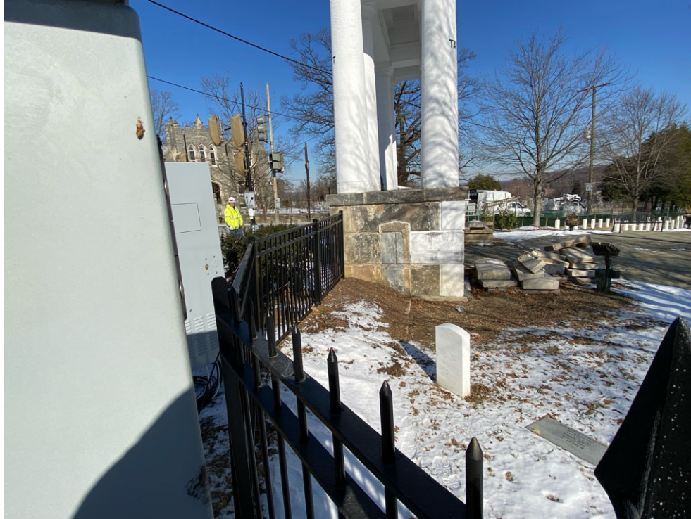
View from the Harewood Rd NW sidewalk adjacent the boundary fence looking north toward the SAHNC Main Entrance Gate. Note temporary aluminum fencing connected to western face and ghost of the outline of the southern wing wall on the stone base (2024).
