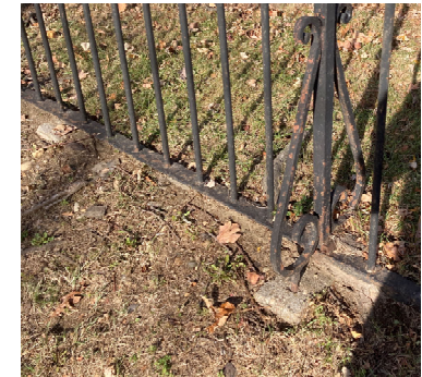
Photo of typical concrete fence post footer (right) and intermediate fence support (left).
